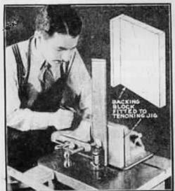
The circular naw tenening liq can be used to good advantage for many shaper operations.
